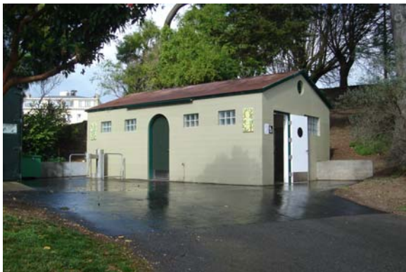
Alta Plaza Restrooms
